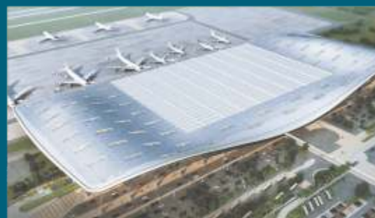
Navi Mumbai International Airport
